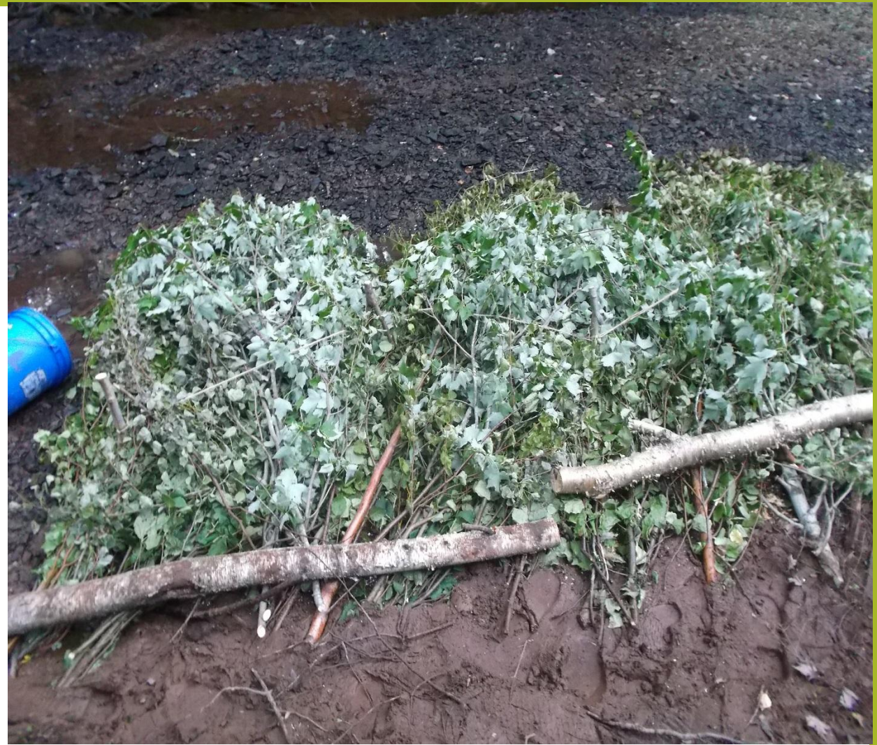
Canfield Creek, Second Brush Mat. The purpose of this installation was to catch sediment when a spring or fall freshet occurs. This is a long term experiment
