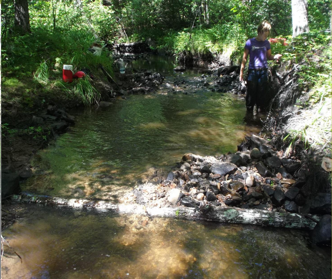
• Patton Brook, Digger Log. Replaced a digger log that was not functioning properly.
