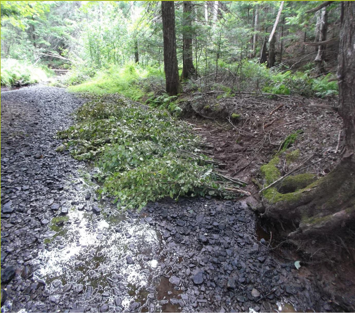
Canfield Creek, Second Brush Mat. The purpose of this installation was to catch sediment when a spring or fall freshet occurs. This is a long term experiment
